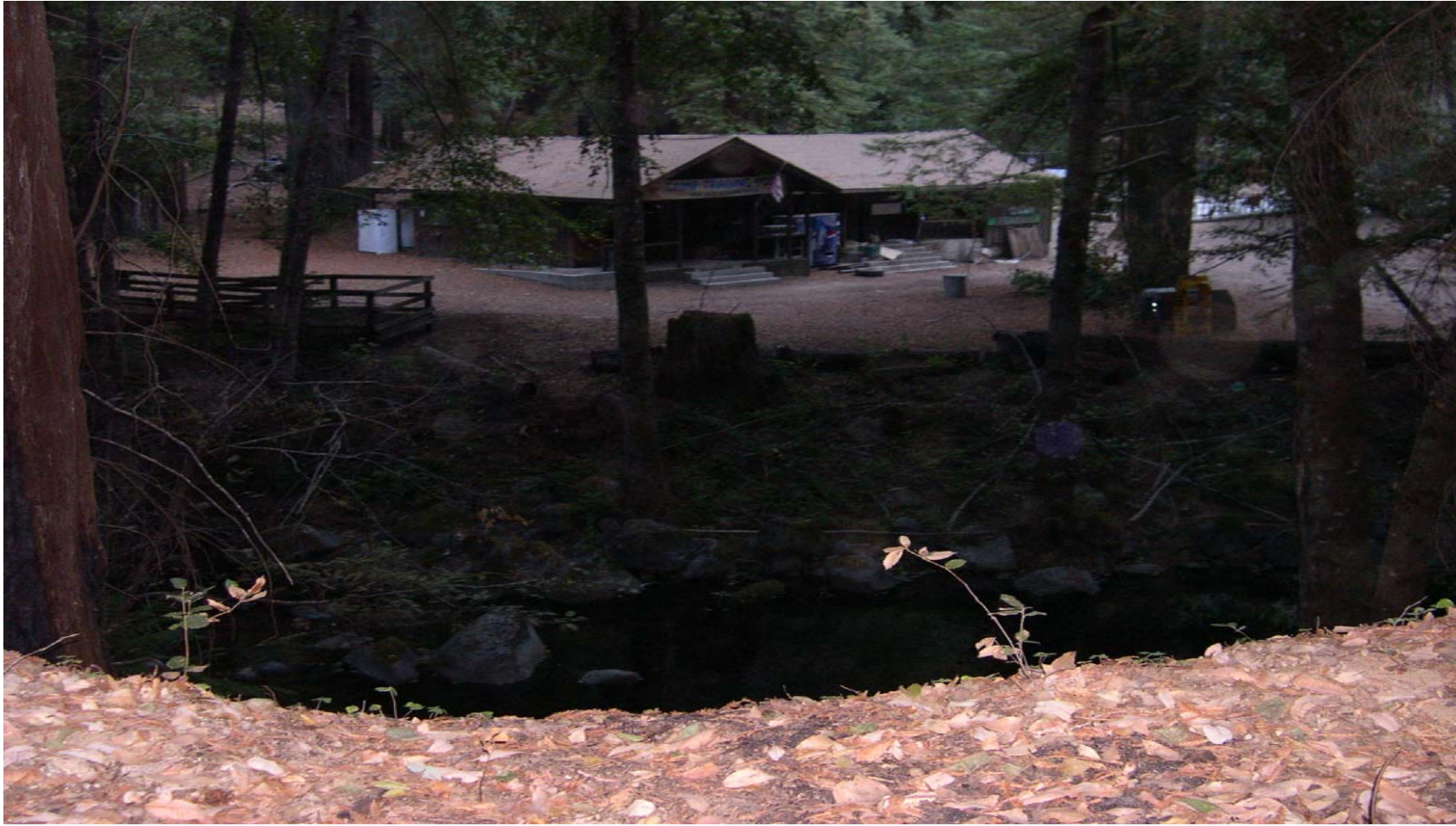
Figure 5: Pico Blanco Boy Scout Camp, camp outpost and store with Little Sur River channel in foreground. This building has the highest probability of flooding of all of the large structures in the camp. It is located on the inside of a short river bend and the bulk of flood energy is focused on the bank opposite of the building. The development of the camp has confined the channel along this reach, note the steep stream banks.
