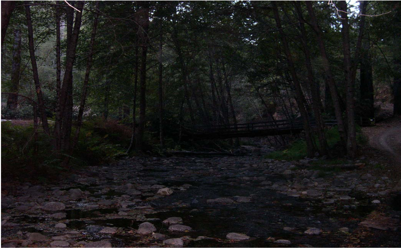
Figure 6: Little Sur River and camp foot bridge at Pico Blanco Boy Scout camp and access road low water ford. Bridge is a potential constriction point for large wood debris at bridge and may cause flows to flood terrace to the left of bridge. Building shown in Figure 5 (store) is to the left of the footbridge in photo. Channel banks have been built up as result of the camp development.
