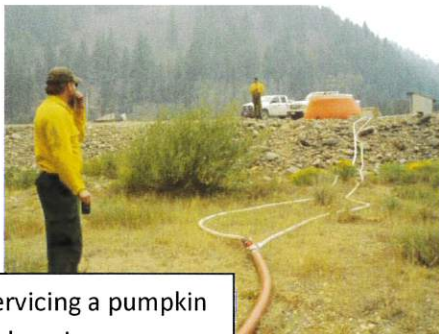
This setup had a 2-inch line running back to a hardened site that trucks could hook up to, fire up the pump, and fill >50 feet from the creek.
