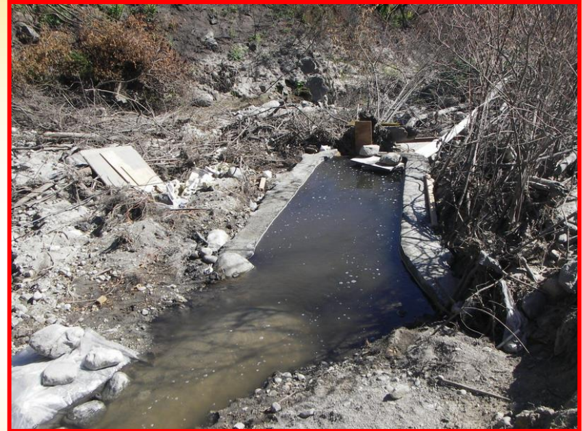
Small diversion structure on Chiliwist Creek
