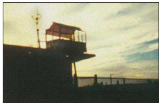
FIGURE 11-1 West Yellowstone Temporary Tower, 1988
