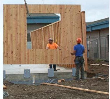
Cross laminated timber project building at Greywolf Elementary in the Sequim School District.
