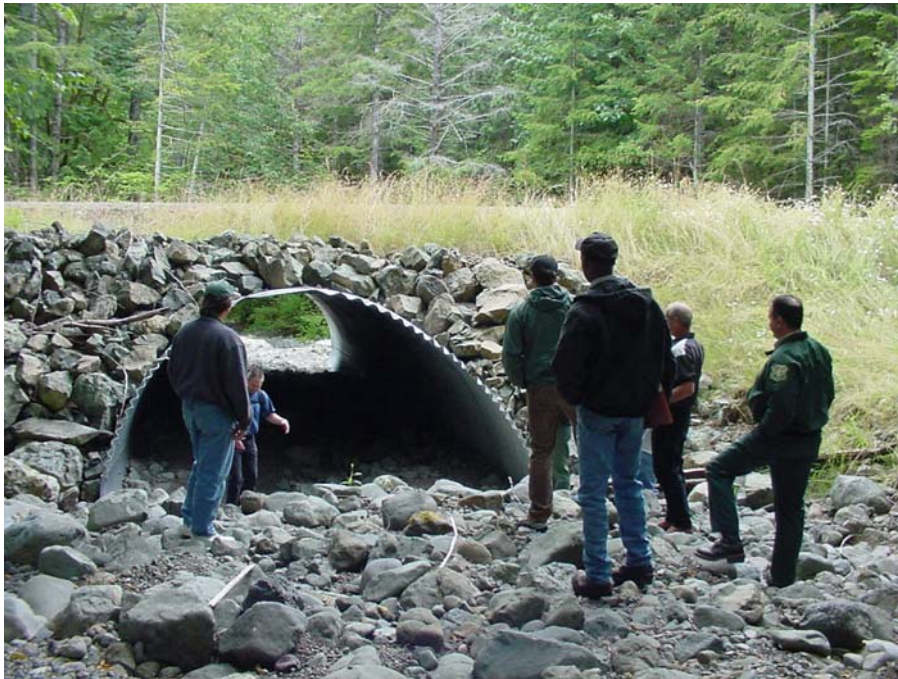
Culvert, fish passage and barrier information was ranked as the 8 th most important data issue. Photograph by David Baker of an in-stream structure (culvert) to abate seasonal instream passage problem, Olympic Province
