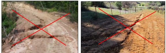
There are a number of solutions to this but the most common is the installation of **waterbars**. Waterbars **DIVERT** water off the feature.
