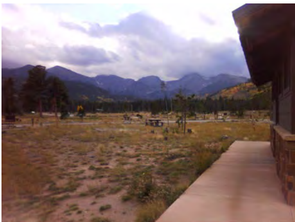
ROMO_31756_B-0379-N Comfort Station GBCG_A.jpg
