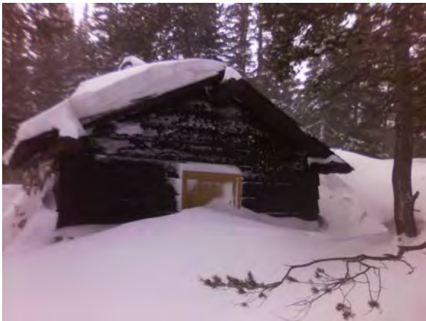
ROMO_31115_B-0157-H Generator Building Bear Lake_B.jpg
