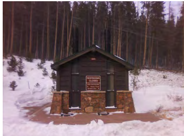
ROMO_74464_B-1121-N Vault Toilet, Bierstadt Trailhead_A.jpg
