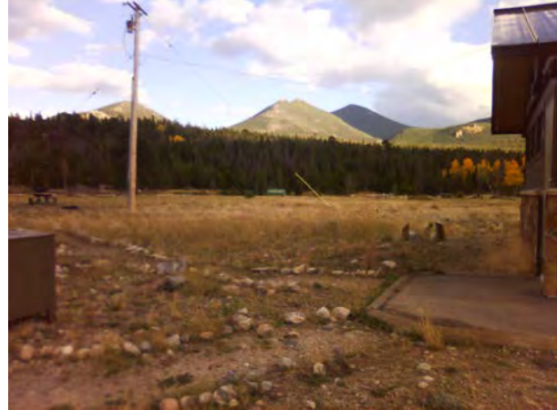
ROMO_31757_B-0408-N Comfort Station GBCG_D.jpg
