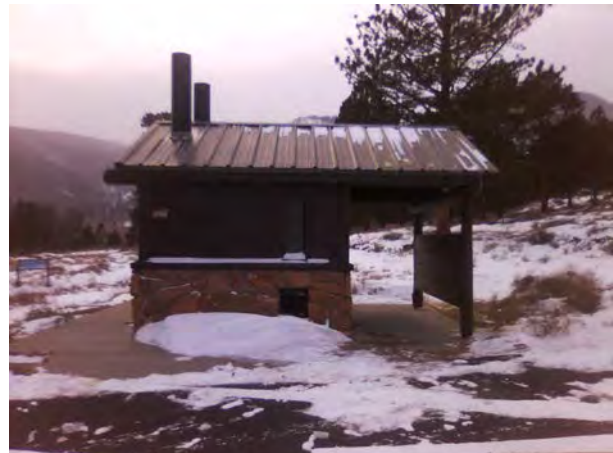
ROMO_60685_B-1053 Hollowell Vault Toilet_A.jpg
