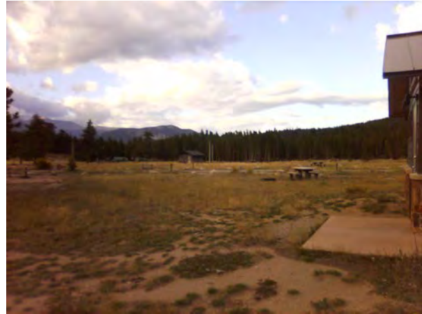
ROMO_31755_B-0378-N Comfort Station GBCG_D.jpg
