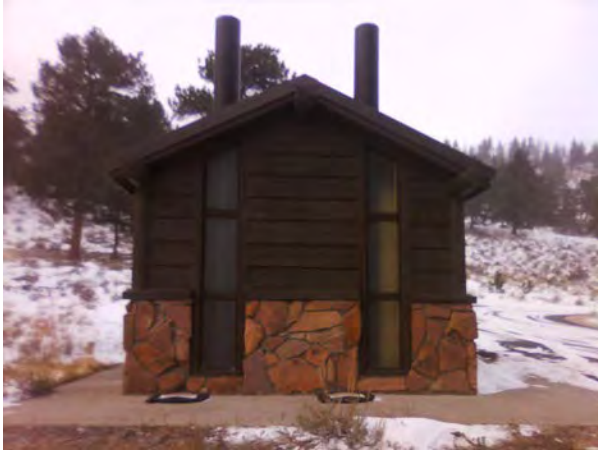
ROMO_60685_B-1053 Hollowell Vault Toilet_D.jpg
