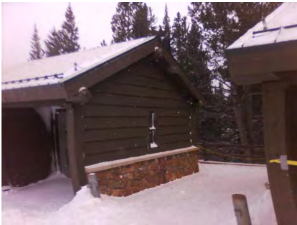
ROMO_82311_B-1125-N Vault Toilet Bear Lake East_B.jpg
