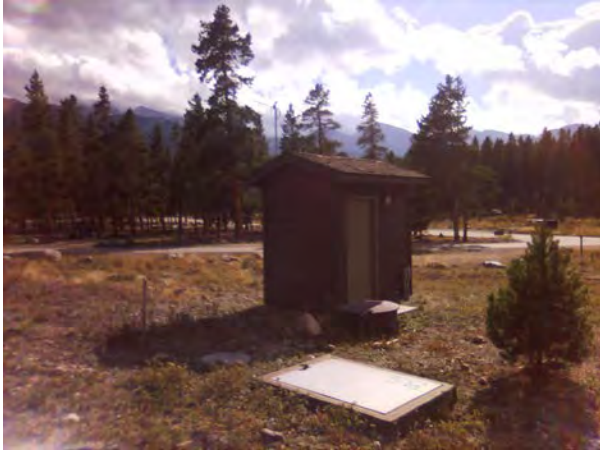
ROMO_31768_B-0994-N Lift Station Control Building_Front2.jpg
