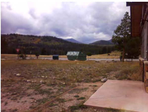
ROMO_31751_B-0374-N Comfort Station GBCG_A.jpg
