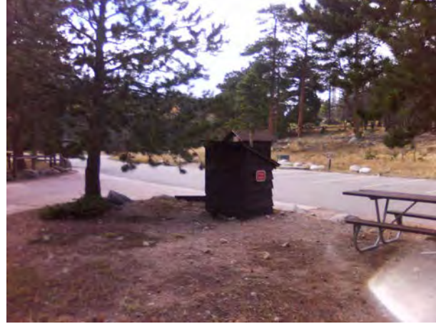
ROMO_31745_B-0184-H Hose House, Glacier Basin Campground_Front.jpg
