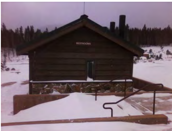
ROMO_82306_B-1119-N Vault Toilet Park & Ride_B.jpg
