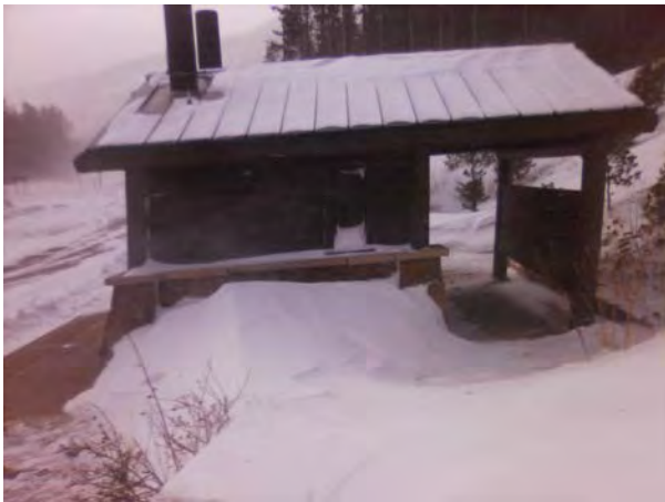
ROMO_74464_B-1121-N Vault Toilet, Bierstadt Trailhead_B.jpg
