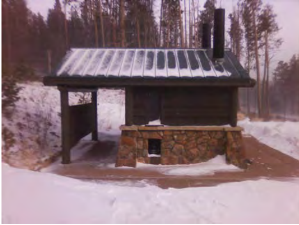
ROMO_74464_B-1121-N Vault Toilet, Bierstadt Trailhead_D.jpg
