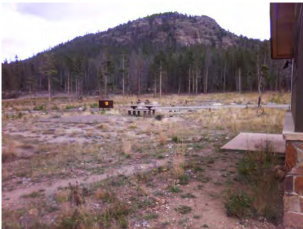
ROMO_31753_B-0376-N Comfort Station GBCG_A.jpg
