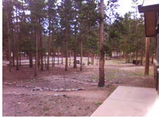
ROMO_31750_B-0373-N Comfort Station GBCG_D.jpg
