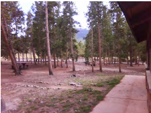
ROMO_31750_B-0373-N Comfort Station GBCG_A.jpg
