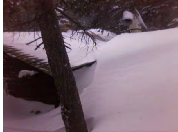
ROMO_31115_B-0157-H Generator Building Bear Lake_C.jpg
