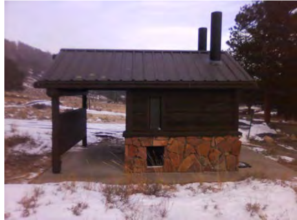
ROMO_60685_B-1053 Hollowell Vault Toilet_C.jpg
