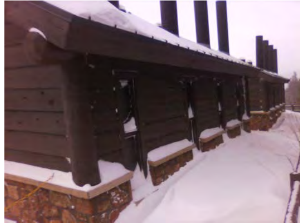
ROMO_82314_B-1126-N Vault Toilet Bear Lake West_C.jpg
