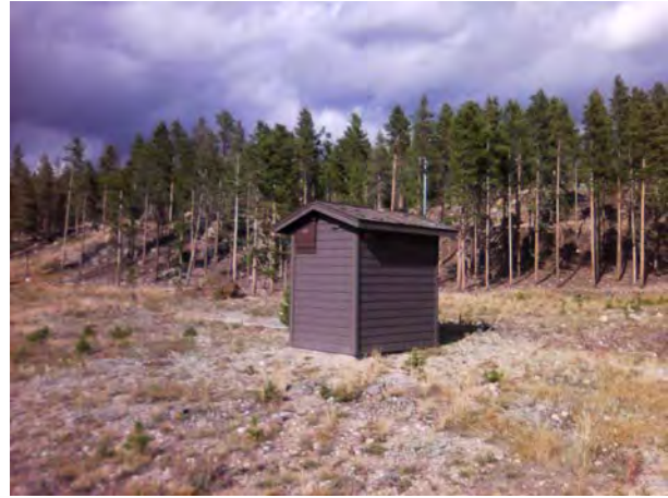
ROMO_31768_B-0994-N Lift Station Control Building_Front.jpg
