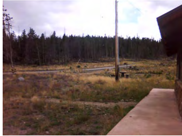
ROMO_31753_B-0376-N Comfort Station GBCG_D.jpg
