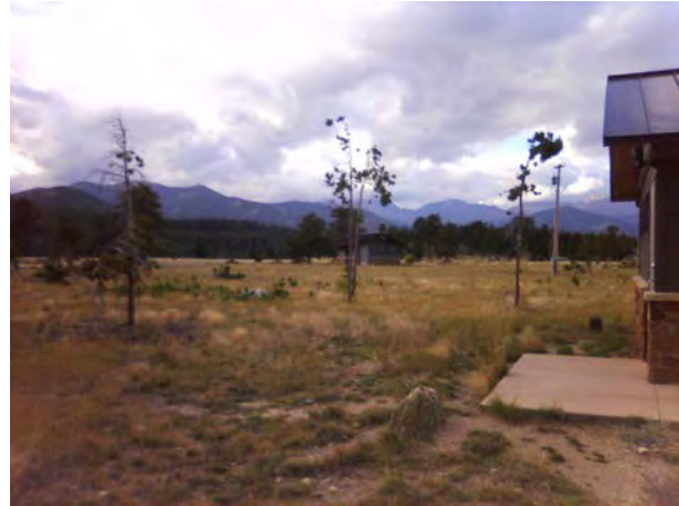
ROMO_31756_B-0379-N Comfort Station GBCG_D.jpg
