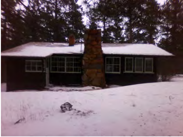
ROMO_31729_Q-0037-H S 3-Bedroom House 00000037_D.jpg
