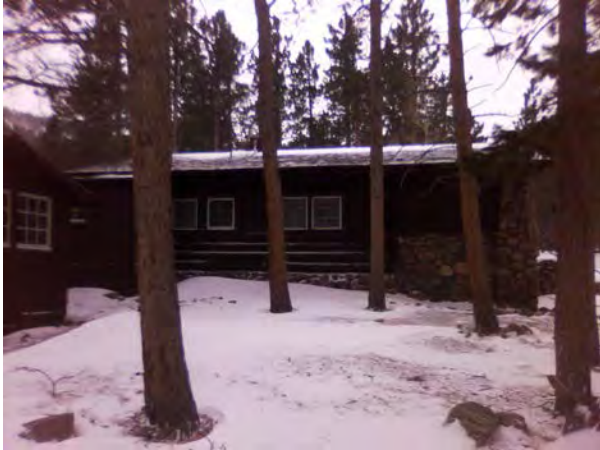
ROMO_31726_B-0036-H Mill Creek Ranger Station_D.jpg
