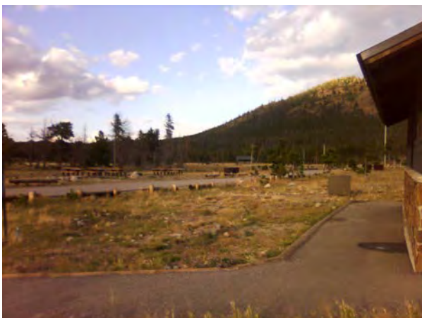
ROMO_31757_B-0408-N Comfort Station GBCG_A.jpg
