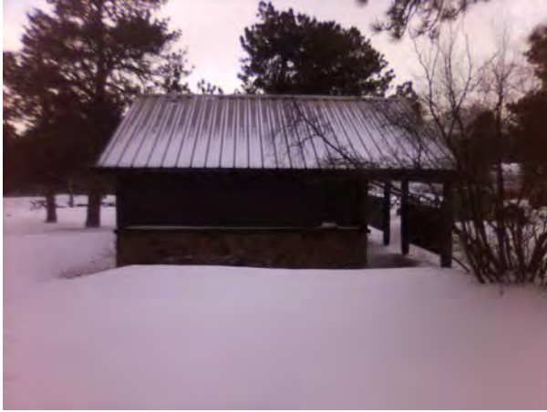
ROMO_31815_B-1054-N Comfort Station, Sprague Lake_D.jpg
