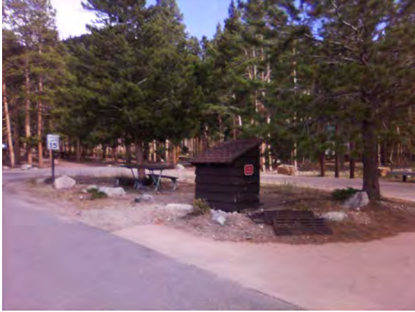
ROMO_31745_B-0184-H Hose House, Glacier Basin Campground_Front2.jpg
