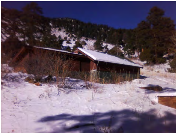
ROMO__Drinking water supply_B.jpg
