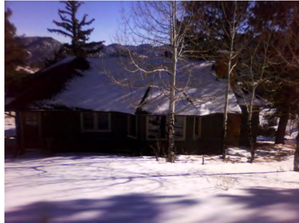
ROMO_30953_Q-0718-H S 4-Bedroom House, Johnston 00000718_C.jpg
