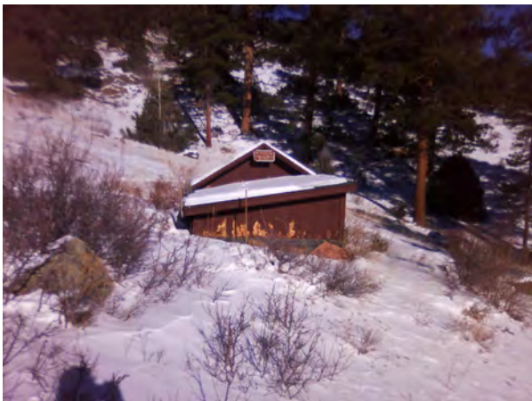
ROMO__Drinking water supply_A.jpg
