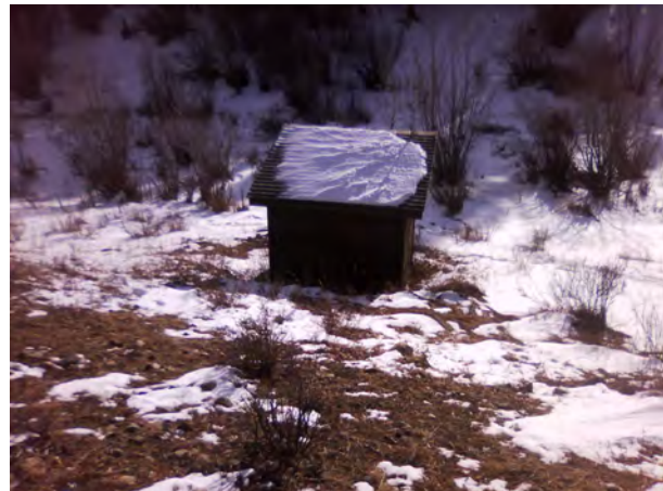
ROMO_98020_B-0603-N Pumphouse, BME_A.jpg
