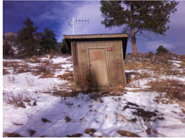
ROMO_98020_B-0603-N Pumphouse, BME_C.jpg
