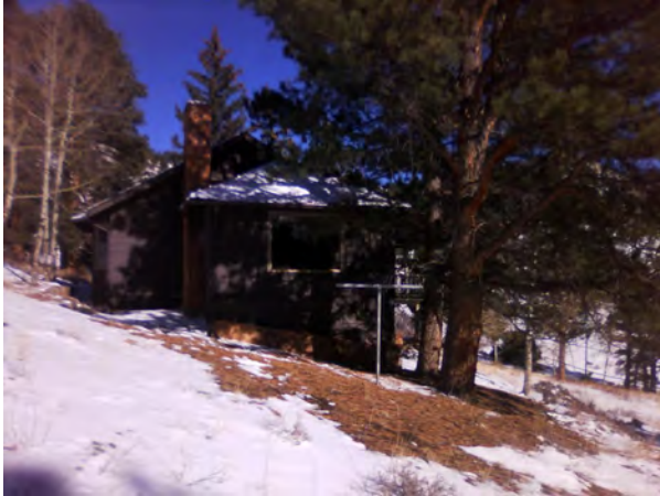
ROMO_30953_Q-0718-H S 4-Bedroom House, Johnston 00000718_D.jpg
