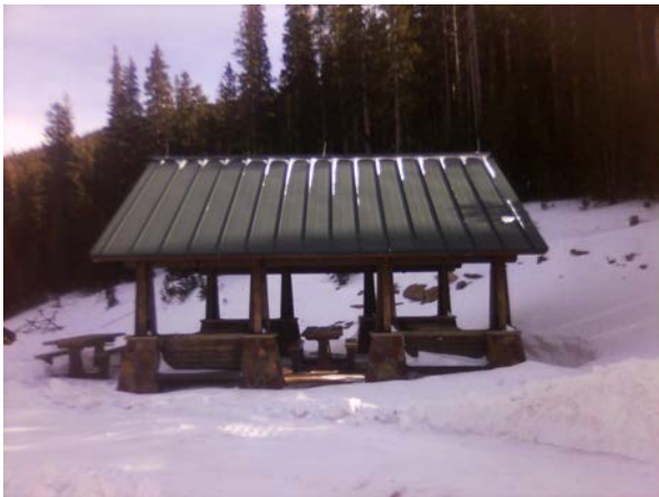
ROMO_82278_B-1127 Picnic Shelter, Hidden Val Picnic_B.jpg
