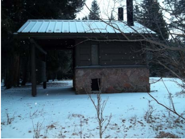
2013_ROMO_25431_B-1056-N Vault Toilet Endovalley South Picnic Area_D.jpg
