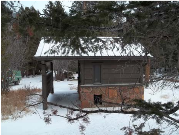
ROMO_25429_Vault Toilet Endo Valley N-Picnic Area (B).JPG
