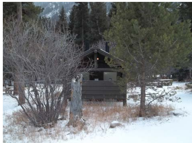
2013_ROMO_25429_B-1055-N Vault Toilet Endovalley North Picnic Area_A.jpg
