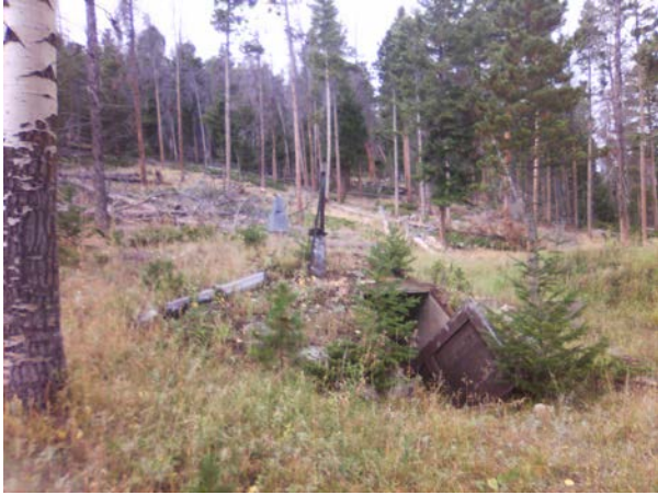
ROMO_25490_B-0985-N Generator Shed Little Horseshoe Park_Front2.jpg
