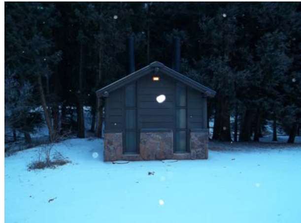
2013_ROMO_25431_B-1056-N Vault Toilet Endovalley South Picnic Area_A.jpg
