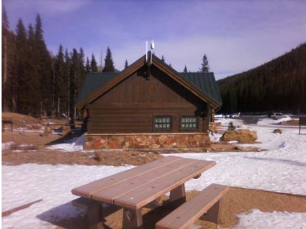
ROMO_69688_B-1093-N Restroom Multi-use Building_D.jpg
