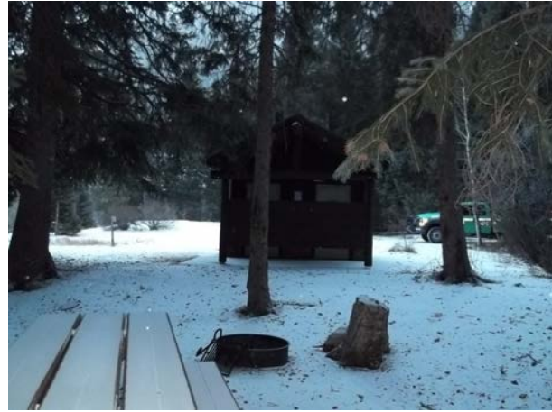
2013_ROMO_25431_B-1056-N Vault Toilet Endovalley South Picnic Area_C.jpg
