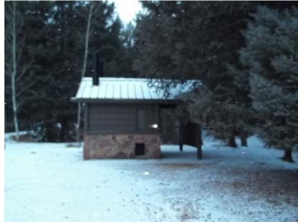
2013_ROMO_25429_B-1055-N Vault Toilet Endovalley North Picnic Area_D.jpg
