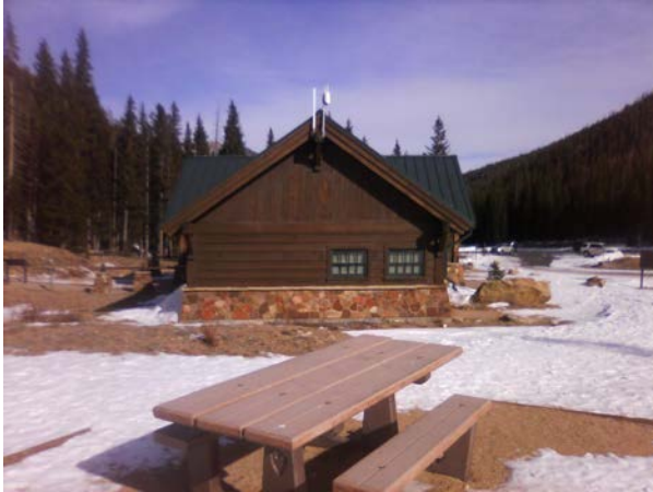
ROMO_69688_B-1093-N Restroom Multi-use Building_D.jpg
