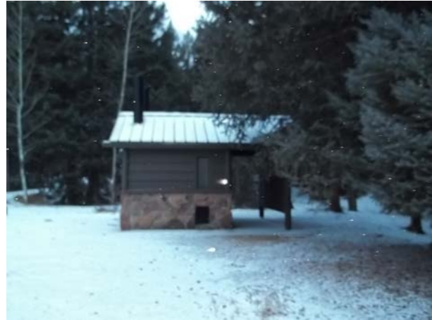
2013_ROMO_25429_B-1055-N Vault Toilet Endovalley North Picnic Area_D.jpg
