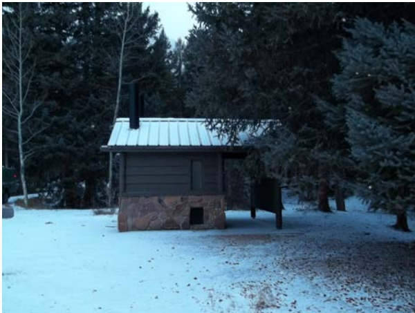
2013_ROMO_25431_B-1056-N Vault Toilet Endovalley South Picnic Area_B.jpg
