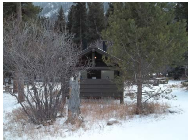
2013_ROMO_25429_B-1055-N Vault Toilet Endovalley North Picnic Area_A.jpg
