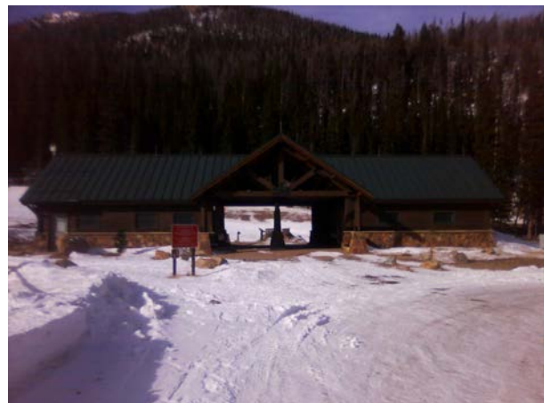
ROMO_69688_B-1093-N Restroom Multi-use Building_A.jpg
