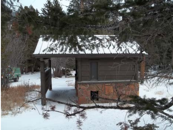
ROMO_25429_Vault Toilet Endo Valley N-Picnic Area (B).JPG
