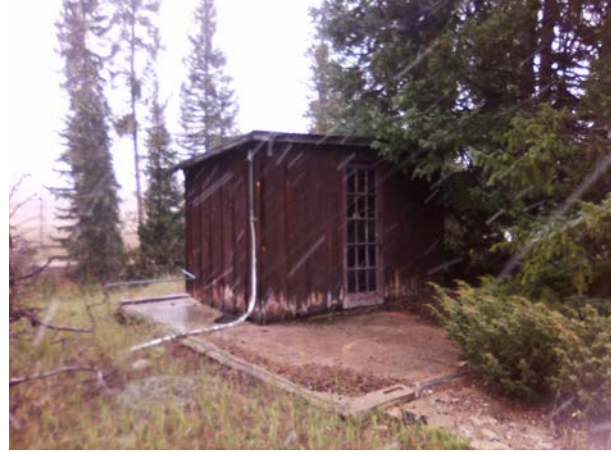
ROMO_14760_B-0725-H Pumphouse "Nelson", Green Mountain_Front.jpg
