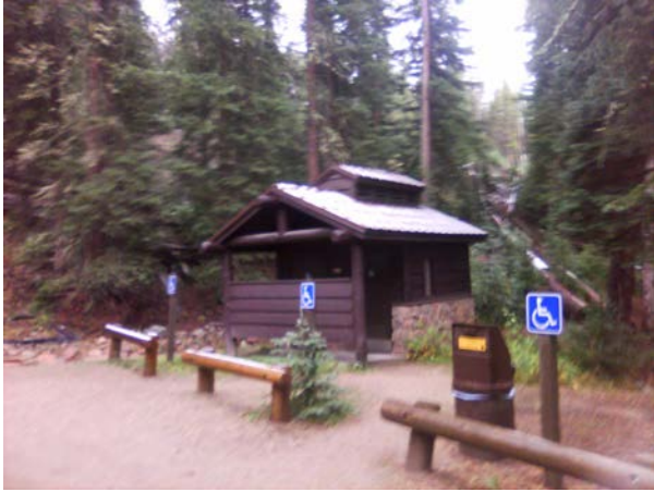
ROMO_14777_B-1050-N Vault Toilet - Coyote Valley_Front.jpg
