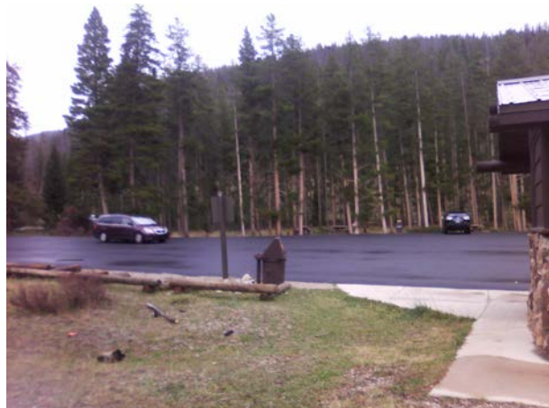
ROMO_14787_B-1069-N Vault Toilet (SST) NSR_B.jpg
