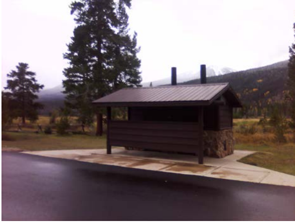
ROMO_14787_B-1069-N Vault Toilet (SST) NSR_Front.jpg
