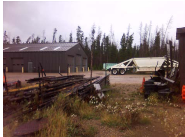
ROMO_37098_B-0187-N Storage Shed, Harbison_B.jpg
