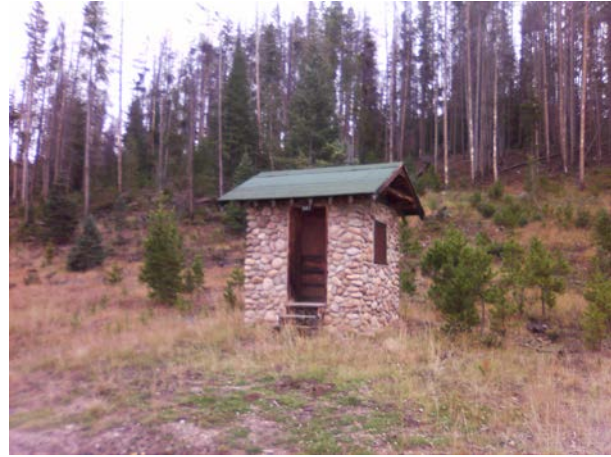
ROMO_97834_B-0587-H Pumphouse - Rock - Green Mountain INACTIVE_Front.jpg
