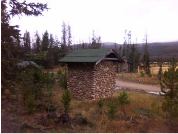
ROMO_97834_B-0587-H Pumphouse - Rock - Green Mountain INACTIVE_Front2.jpg
