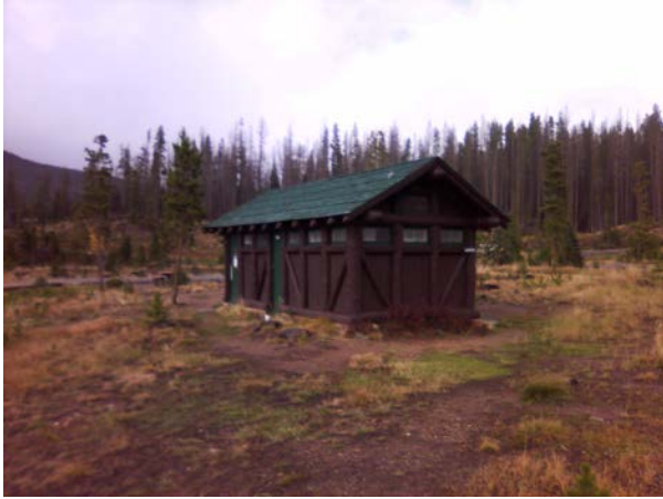
ROMO_14817_B-0246-H Comfort Station, Log Second A Loop_Front.jpg
