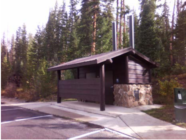
ROMO_14770_B-1048-N Vault Toilet (SST) Green Mountain_Front.jpg
