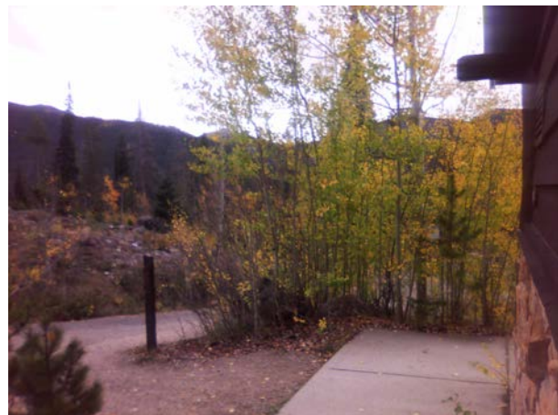
ROMO_14697_B-1034-N Vault Toilet - North Inlet_B.jpg
