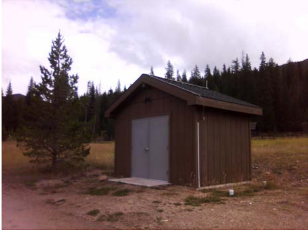
ROMO_97831_B-0867-N Pumphouse, Green Mountain ACTIVE (old #346)_Front.jpg
