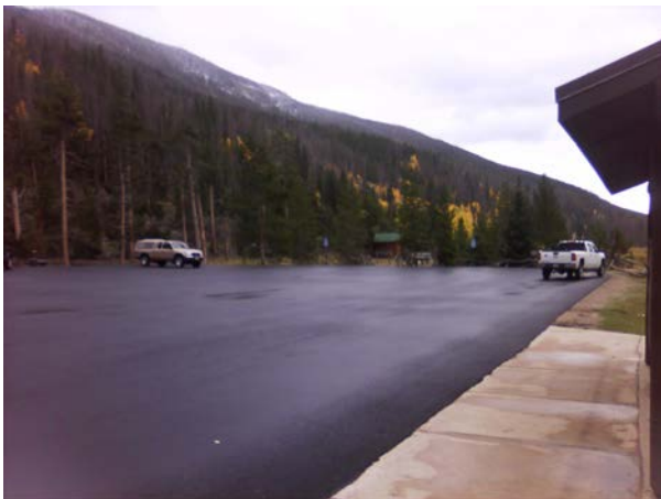
ROMO_14787_B-1069-N Vault Toilet (SST) NSR_A.jpg
