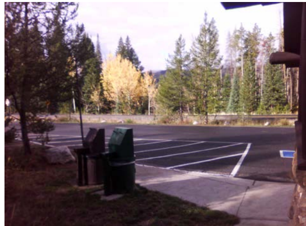
ROMO_14770_B-1048-N Vault Toilet (SST) Green Mountain_B.jpg
