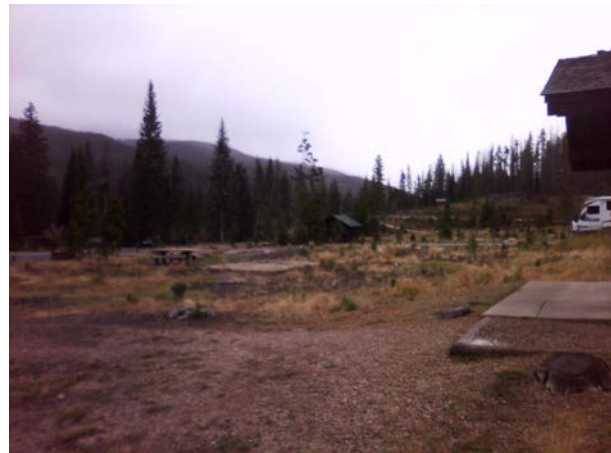
ROMO_14826_B-0352-N Comfort Station, Brick B Loop_B.jpg
