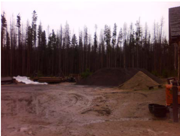
ROMO_14813_B-0241-H Historic Barn (Timber Creek Road Camp)_A.jpg
