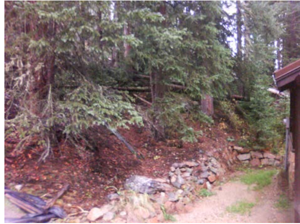
ROMO_14777_B-1050-N Vault Toilet - Coyote Valley_D.jpg
