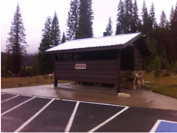
ROMO_39408_B-1091-N Vault Toilet, SST, Bowen-Baker_Front.jpg
