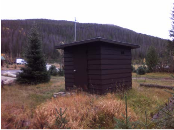
ROMO_97840_B-0689-N Pumphouse with chlorinator TCCG_Front2.jpg
