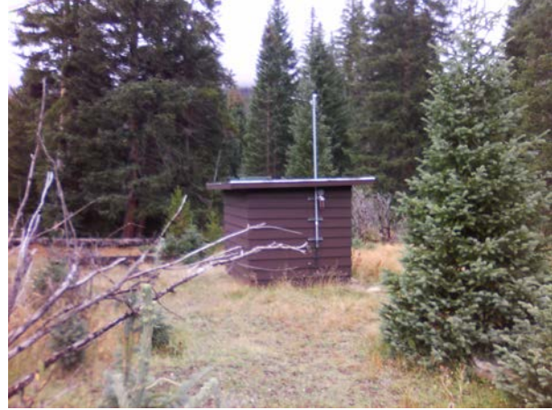
ROMO_97840_B-0689-N Pumphouse with chlorinator TCCG_Front.jpg
