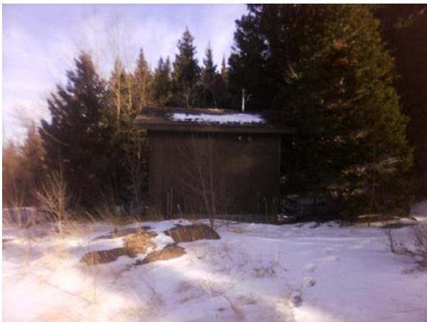
ROMO__Well Pump House east of Lily Lake Visitor Center_A.jpg
