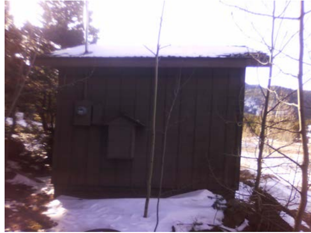
ROMO__Well Pump House east of Lily Lake Visitor Center_C.jpg
