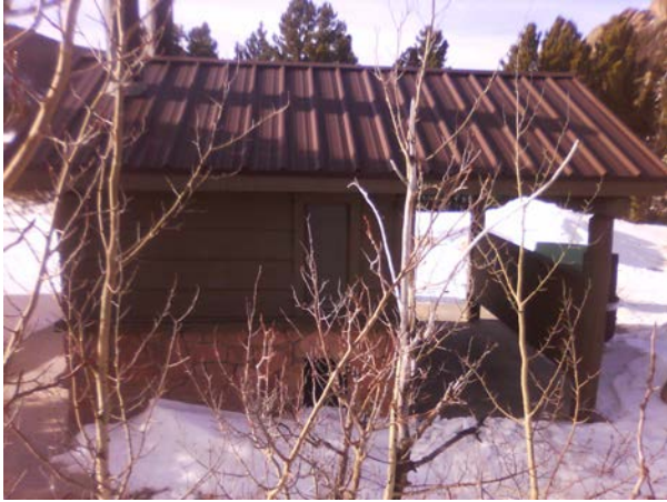
ROMO_85270_B-1129-N Vault Toilet Lily Lake_D.jpg
