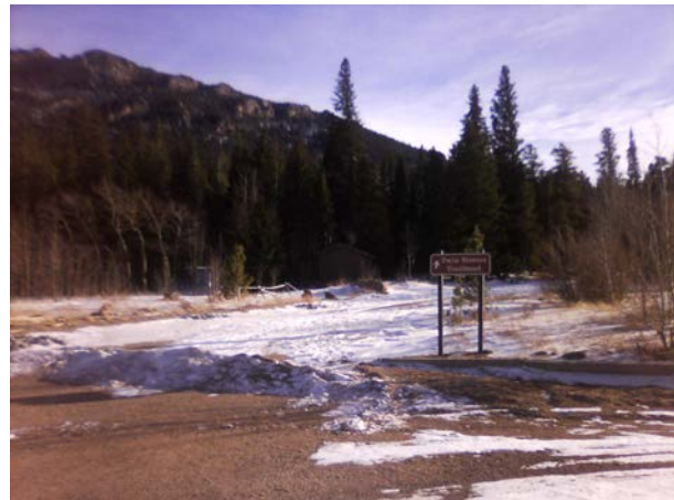
ROMO__Well Pump House east of Lily Lake Visitor Center_A-1.jpg
