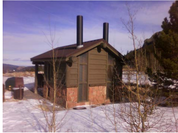
ROMO_85270_B-1129-N Vault Toilet Lily Lake_C.jpg
