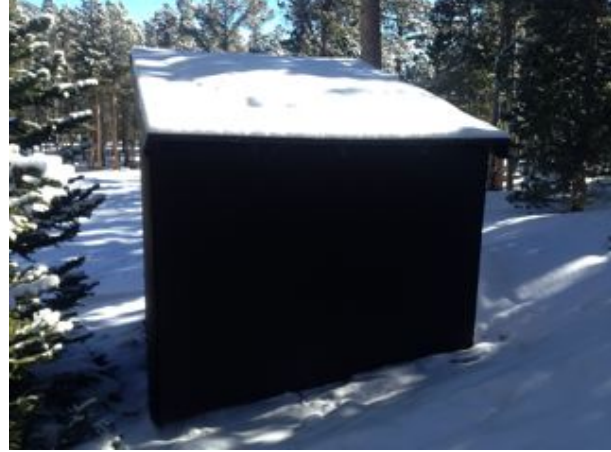
2014_ROMO_23746_B-1058-N Vault Toilet Longs Peak Campground_x.jpg
