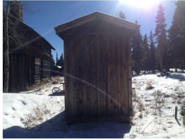
2014_ROMO_98026_B-1025-N Pumphouse, Leiffer_x.jpg
