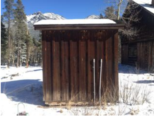
2014_ROMO_98026_B-1025-N Pumphouse, Leiffer_x.jpg
