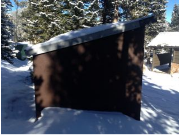
2014_ROMO_23746_B-1058-N Vault Toilet Longs Peak Campground_x.jpg
