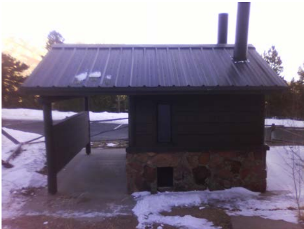
ROMO_23745_B-1057-N Vault Toilet Longs Peak Parking Lot_B.jpg
