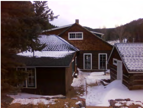
ROMO_25300_B-1000-H Office & Residence - McGraw Ranch_C.jpg
