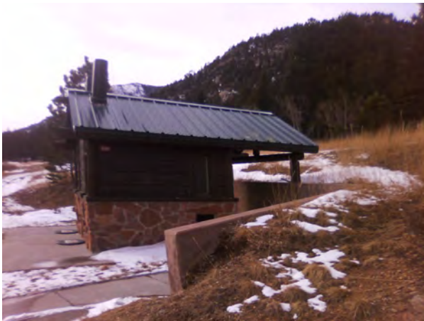
ROMO_37231_B-1066-N Vault Toilet, McGraw Ranch_B.jpg
