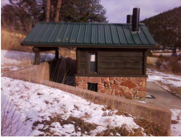
ROMO_37231_B-1066-N Vault Toilet, McGraw Ranch_D.jpg
