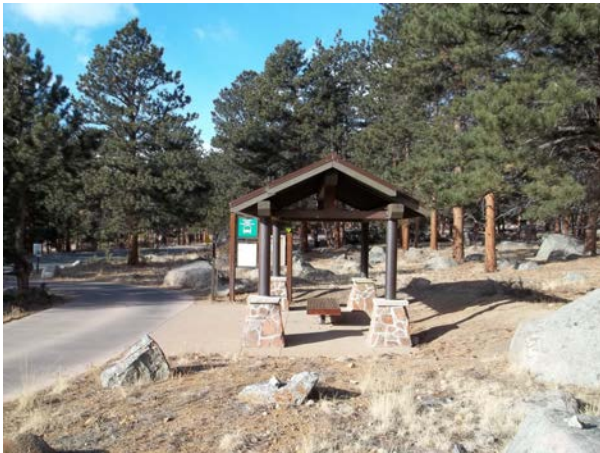
2013_ROMO_106803_B-1136-ESD Bus Shelter Moraine Park Campground_B.jpg
