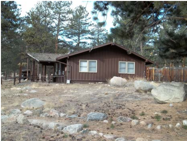
2013_ROMO_31359_B-0619-N Ranger Station, Moraine Park Campground_B.jpg
