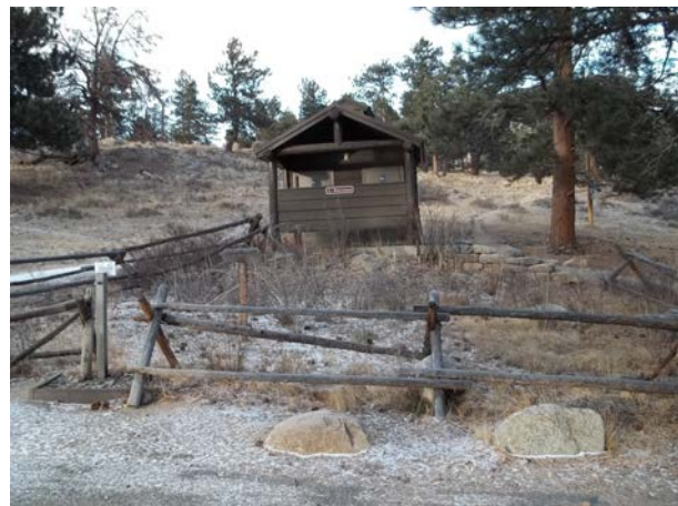
2013_ROMO_37082_B-1032-N Vault Toilet, West Campground MPCG_A.jpg
