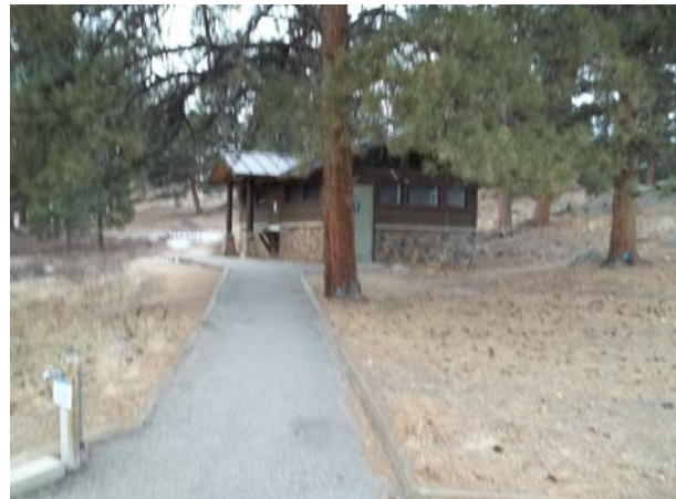
2013_ROMO_31352_B-0613-N Comfort Station MPCG_A.jpg
