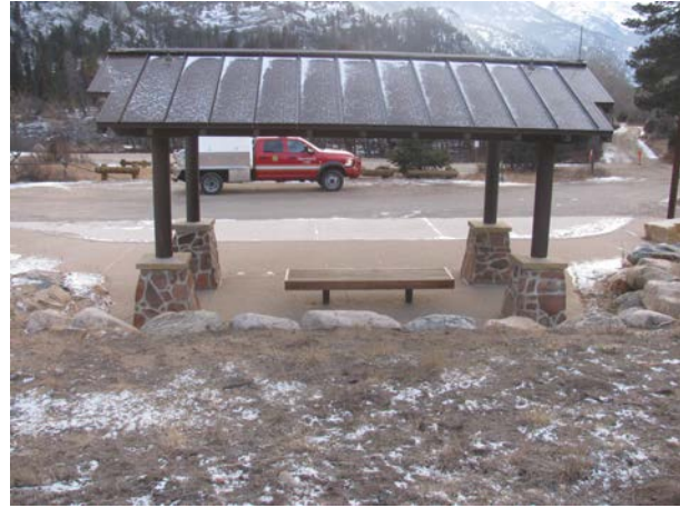
2014_ROMO_106816_B-1137-N Bus Shelter Fern LakeTrailhead_C.jpg
