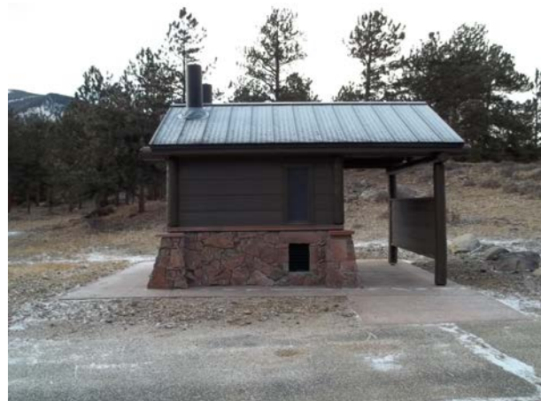
2013_ROMO_Vault Toilet C Loop MPCG_Vault Toilet C Loop MPCG_A.jpg
