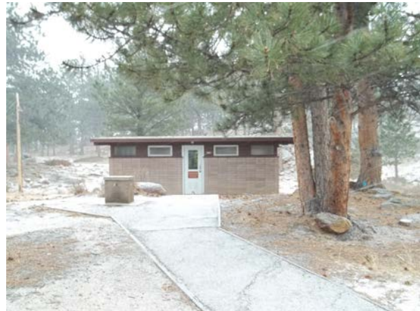
2013_ROMO_31358_B-0618-N Comfort Station, Moraine Park Campground_A.jpg
