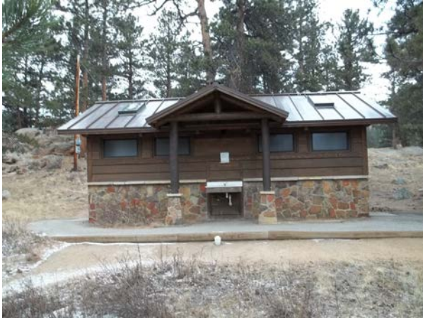
2013_ROMO_31352_B-0613-N Comfort Station MPCG_D.jpg
