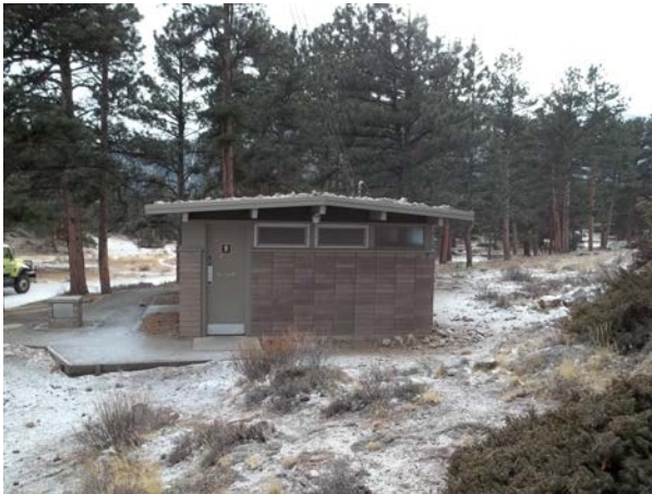
2013_ROMO_31356_B-0616-N Comfort Station, Moraine Park Campground_B.jpg
