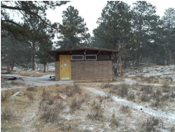
2013_ROMO_31358_B-0618-N Comfort Station, Moraine Park Campground_B.jpg
