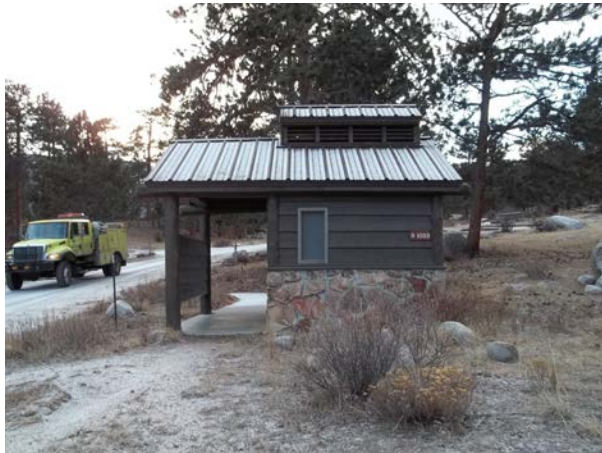
2013_ROMO_37083_B-1033-N Vault Toilet, East Campground MPCG_B.jpg
