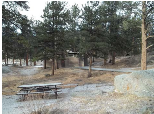
2013_ROMO_31355_B-0615-N Comfort Station, Moraine Park Campground_A.jpg
