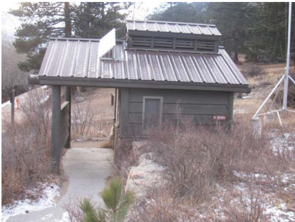
2014_ROMO_37081_B-1030-N Vault Toilet, Cub Lake Trailhead_B.jpg
