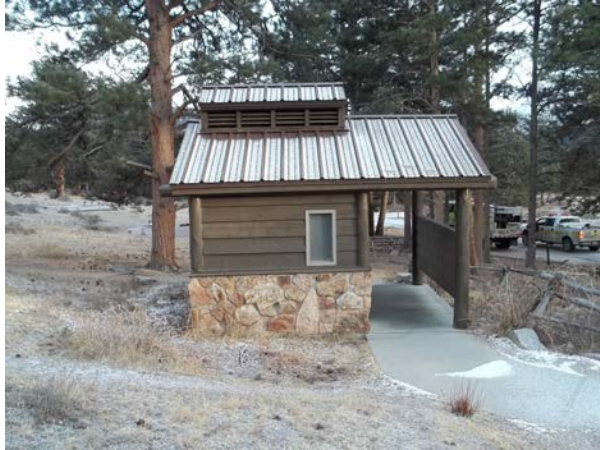
2013_ROMO_37082_B-1032-N Vault Toilet, West Campground MPCG_D.jpg
