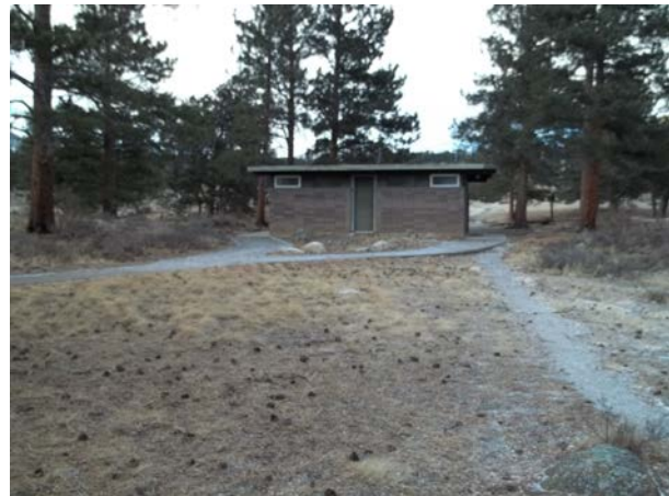
2013_ROMO_31354_B-0614-N Comfort Station MPCG_A.jpg
