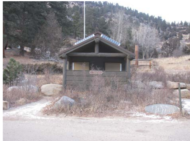
2014_ROMO_37081_B-1030-N Vault Toilet, Cub Lake Trailhead_A.jpg
