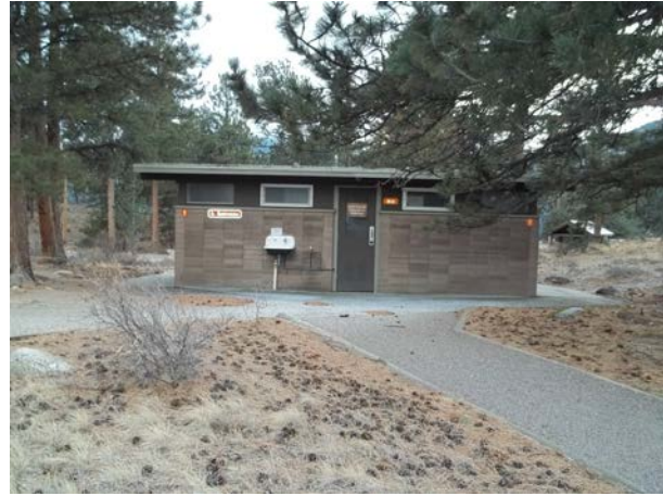
2013_ROMO_31354_B-0614-N Comfort Station MPCG_C.jpg
