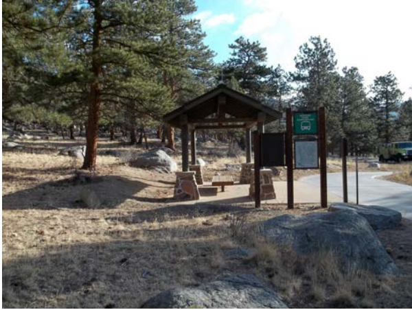
2013_ROMO_106803_B-1136-ESD Bus Shelter Moraine Park Campground_D.jpg
