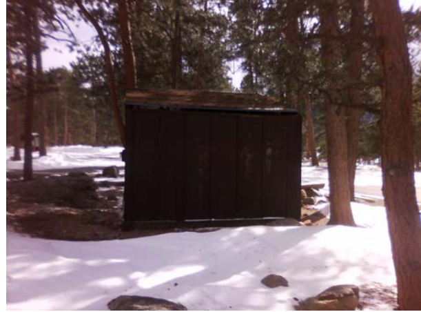
ROMO__BUILDING NEXT TO B-0999_C.jpg
