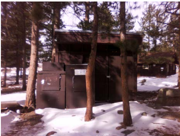
ROMO__BUILDING NEXT TO B-0999_A.jpg
