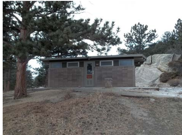
2013_ROMO_31356_B-0616-N Comfort Station, Moraine Park Campground_A.jpg
