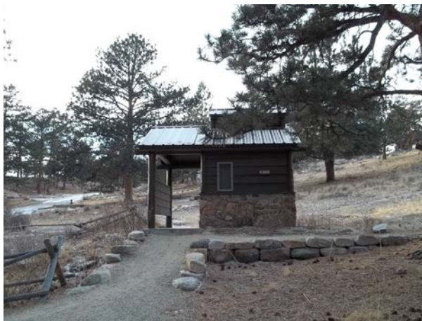
2013_ROMO_37082_B-1032-N Vault Toilet, West Campground MPCG_B.jpg
