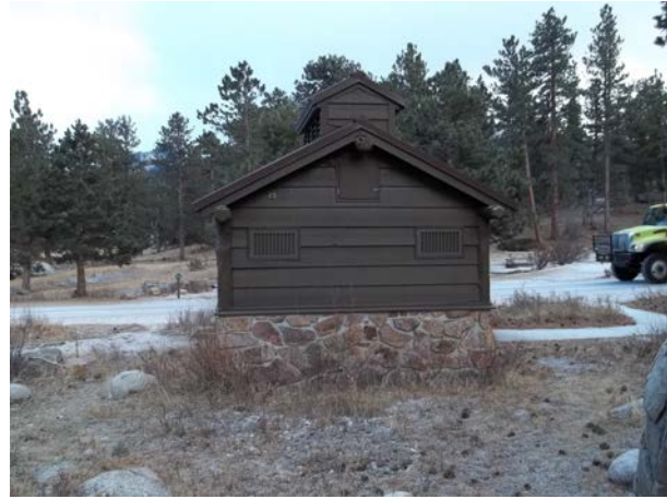
2013_ROMO_37083_B-1033-N Vault Toilet, East Campground MPCG_C.jpg
