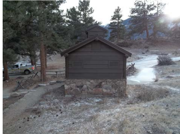
2013_ROMO_37082_B-1032-N Vault Toilet, West Campground MPCG_C.jpg
