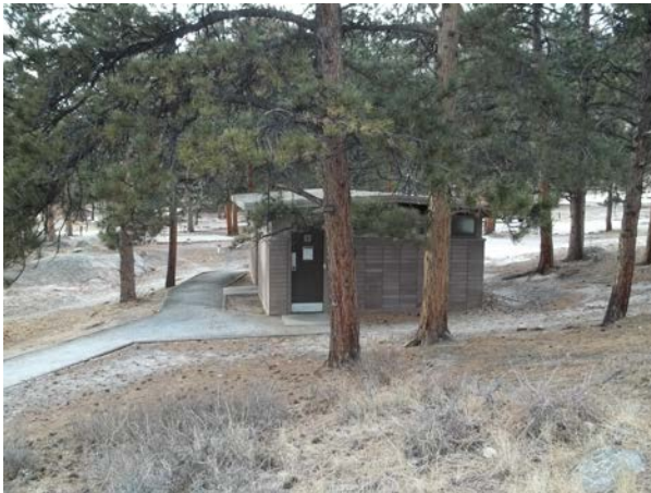
2013_ROMO_31355_B-0615-N Comfort Station, Moraine Park Campground_B.jpg
