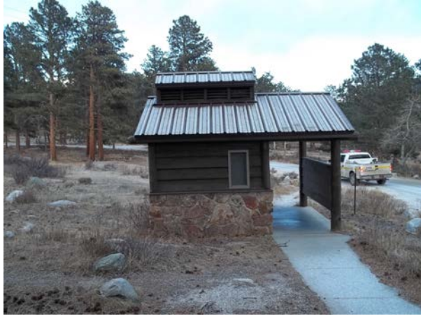
2013_ROMO_37083_B-1033-N Vault Toilet, East Campground MPCG_D.jpg
