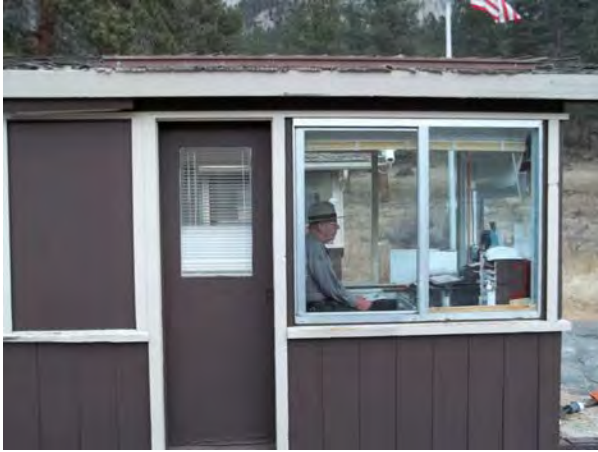
2013_ROMO_24050_B-0670-N Kiosk - Entrance Station Fall River_D.jpg
