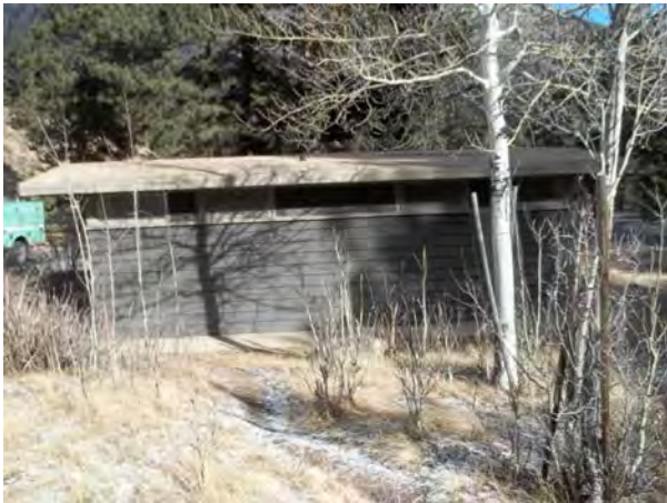
2013_ROMO_25281_B-0367-N Comfort Station Aspenglen Campground_B.jpg
