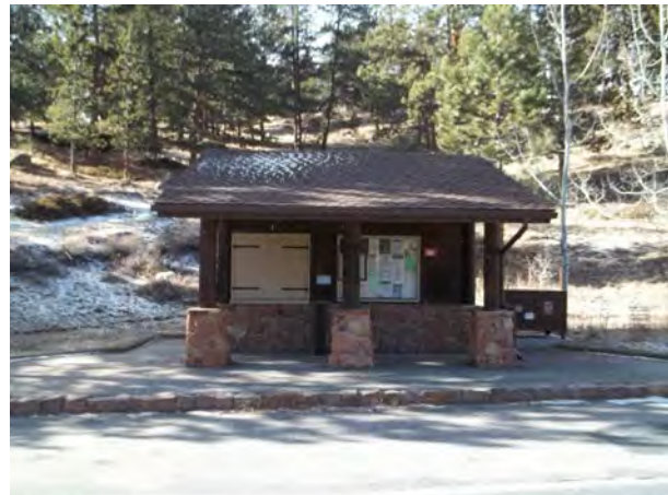
2013_ROMO_25288_B-0992-N Kiosk Aspenglen Campground_A.jpg
