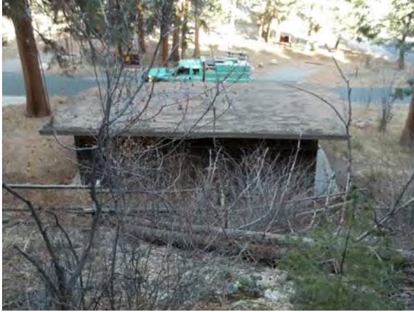
2013_ROMO_25282_B-0401-N Comfort Station Aspenglen Campground_C.jpg
