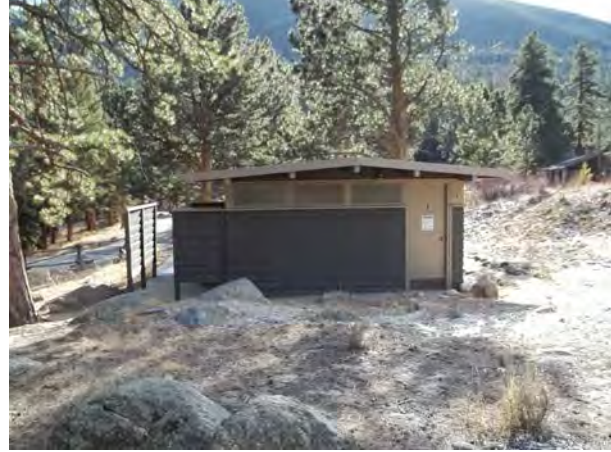
2013_ROMO_25280_B-0366-N Comfort Station Aspenglen Campground_C.jpg
