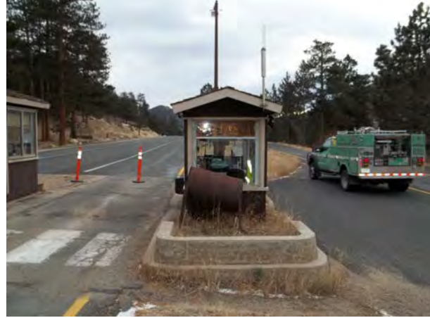
2013_ROMO_24048_B-0669-N Kiosk - Entrance Station Fall River_C.jpg
