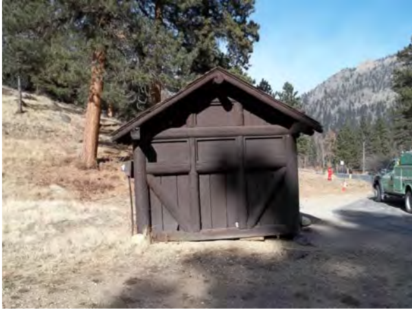
2013_ROMO_Firewood Sales Bldg Aspenglen Campground _Firewood Sales Bldg Aspenglen Campground_D.jpg
