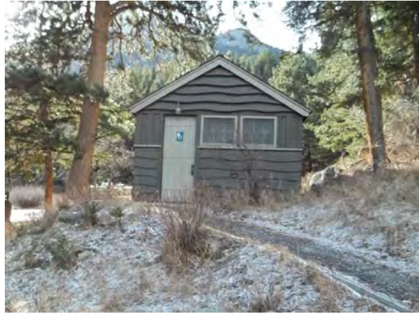
2013_ROMO_25279_B-0153-H Comfort Station Aspenglen Campground_C.jpg
