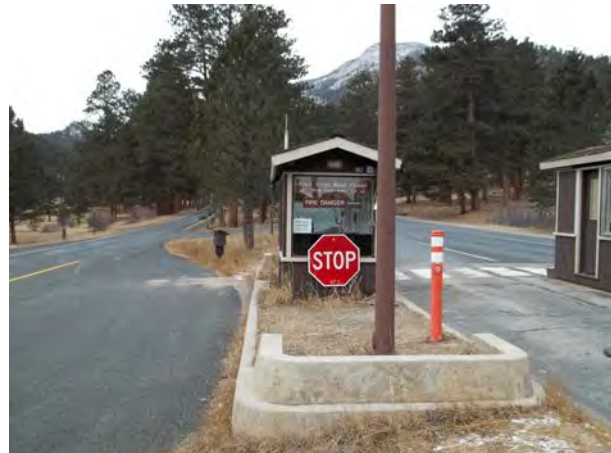
2013_ROMO_24048_B-0669-N Kiosk - Entrance Station Fall River_A.jpg
