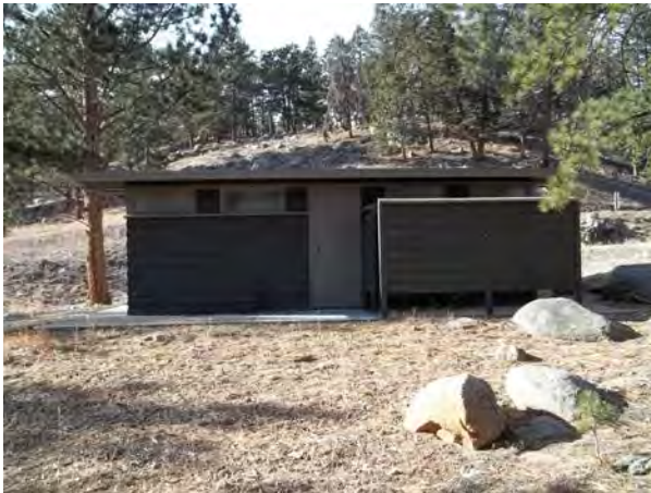
2013_ROMO_25280_B-0366-N Comfort Station Aspenglen Campground_B.jpg
