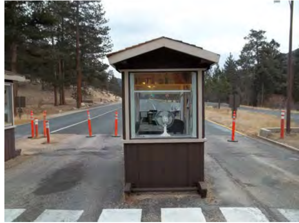
2013_ROMO_24052_B-0671-N Kiosk - Entrance Station Fall River_C.jpg
