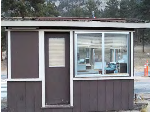
2013_ROMO_24052_B-0671-N Kiosk - Entrance Station Fall River_D.jpg
