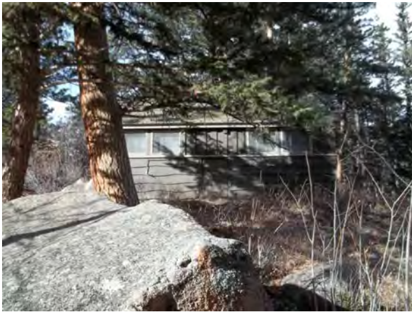
2013_ROMO_25279_B-0153-H Comfort Station Aspenglen Campground_B.jpg
