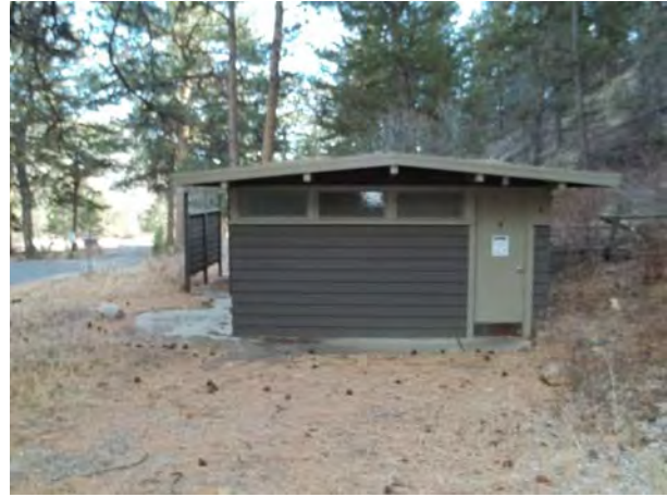
2013_ROMO_25282_B-0401-N Comfort Station Aspenglen Campground_B.jpg
