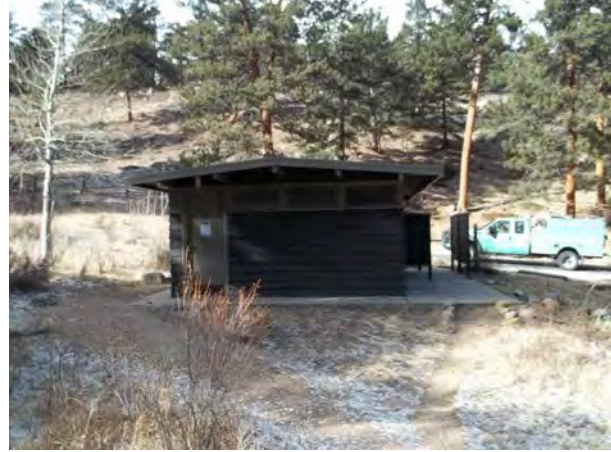
2013_ROMO_25281_B-0367-N Comfort Station Aspenglen Campground_C.jpg
