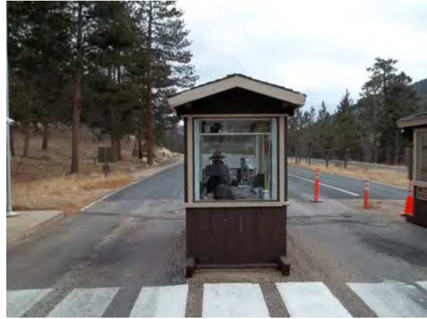
2013_ROMO_24050_B-0670-N Kiosk - Entrance Station Fall River_C.jpg
