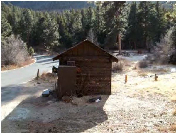
2013_ROMO_Firewood Sales Bldg Aspenglen Campground _Firewood Sales Bldg Aspenglen Campground_B.jpg
