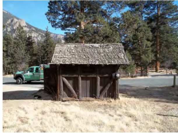
2013_ROMO_Firewood Sales Bldg Aspenglen Campground _Firewood Sales Bldg Aspenglen Campground_C.jpg
