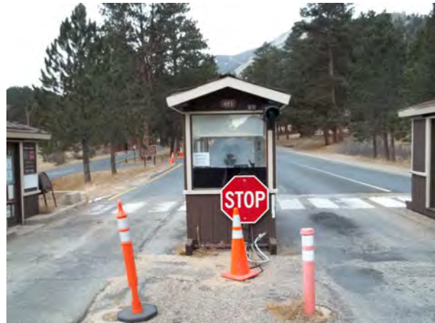
2013_ROMO_24052_B-0671-N Kiosk - Entrance Station Fall River_A.jpg
