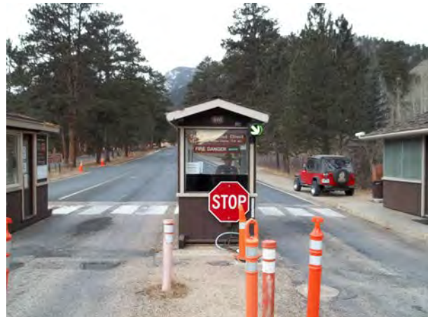
2013_ROMO_24050_B-0670-N Kiosk - Entrance Station Fall River_A.jpg
