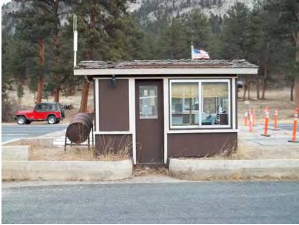
2013_ROMO_24048_B-0669-N Kiosk - Entrance Station Fall River_D.jpg
