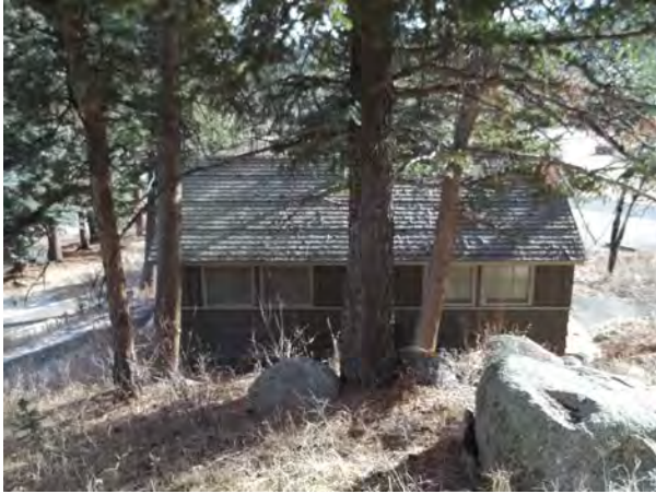
2013_ROMO_25279_B-0153-H Comfort Station Aspenglen Campground_D.jpg
