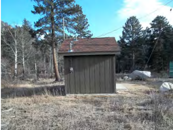
2013_ROMO_98014_B-0688-N Pumphouse, Smith Sisters (Aspenglen)_D.jpg
