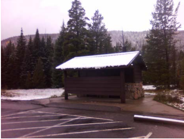
ROMO_37225_B-1092-N Vault Toilet, Colorado River Trailhead_Front.jpg
