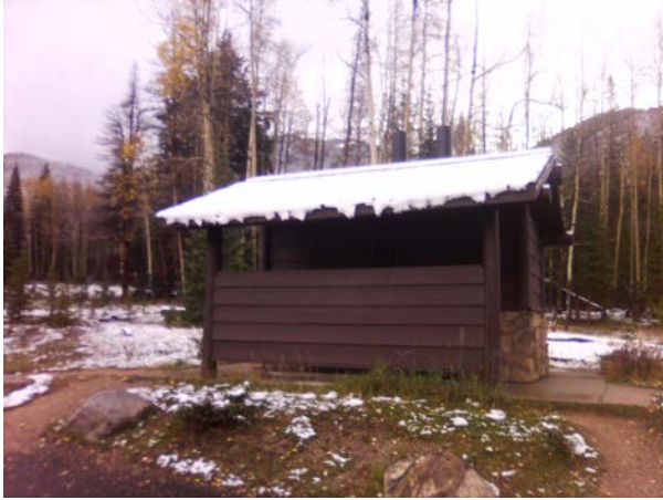
ROMO_45450_B-1087 Vault Toilet, Timber Lake Trailhead_Front.jpg
