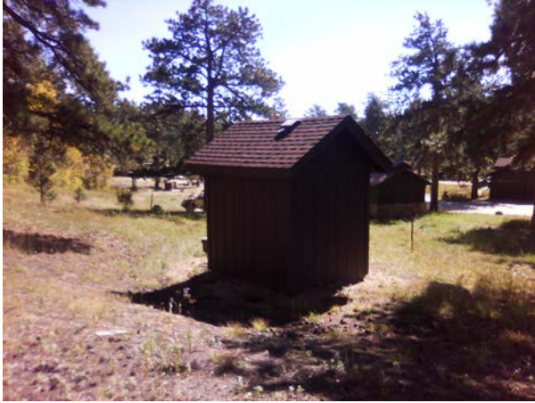
ROMO_98025_B-0987-N Pumphouse - new by Good house_Front2.jpg
