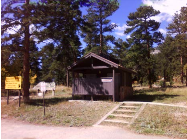
ROMO_23682_B-0996-N Sandbeach TrIHd Vault Toilet_Front.jpg
