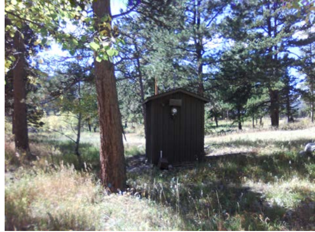
ROMO__WILDBASIN LODGE CISTERN PUMPHOUSE_Front.jpg
