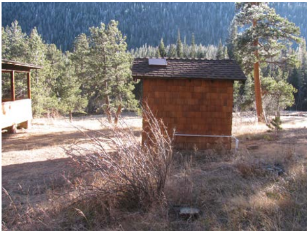
2013_ROMO_98016_B-0851-N Pumphouse, Deer Haven_B.jpg
