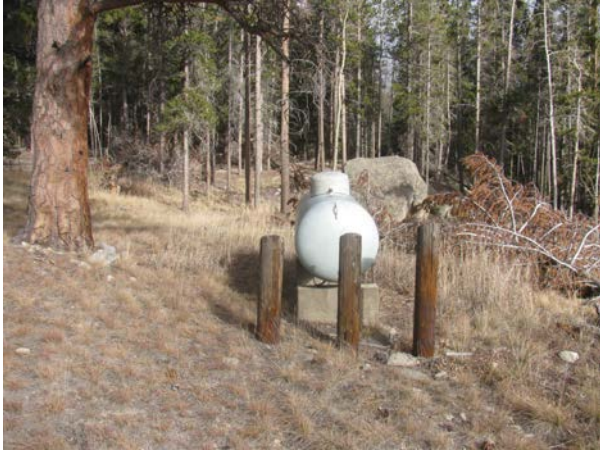
2013_ROMO_Propane Tank Wild Basin_Propane Tank Wild Basin_D.jpg
