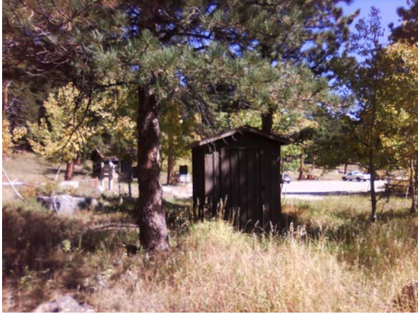
ROMO__WILDBASIN LODGE CISTERN PUMPHOUSE_Front2.jpg
