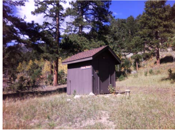
ROMO_98025_B-0987-N Pumphouse - new by Good house_Front.jpg
