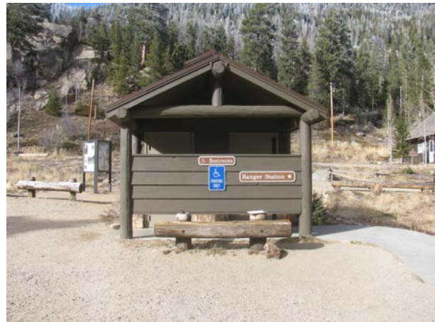
2013_ROMO_23683_B-1035-N Wild Basin Vault Toilet_A.jpg
