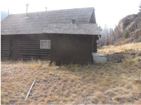
2013_ROMO_23677_B-0819-N Tackroom/Storage @ Ranger Station_B.jpg
