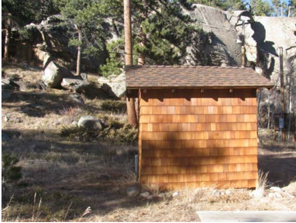
2013_ROMO_98016_B-0851-N Pumphouse, Deer Haven_D.jpg
