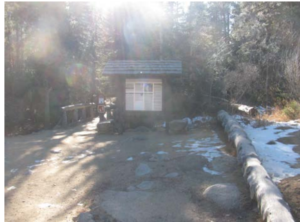
2013_ROMO_Wild Basin Kiosk E. Parking Lot_Wild Basin Kiosk E. Parking Lot_A.jpg
