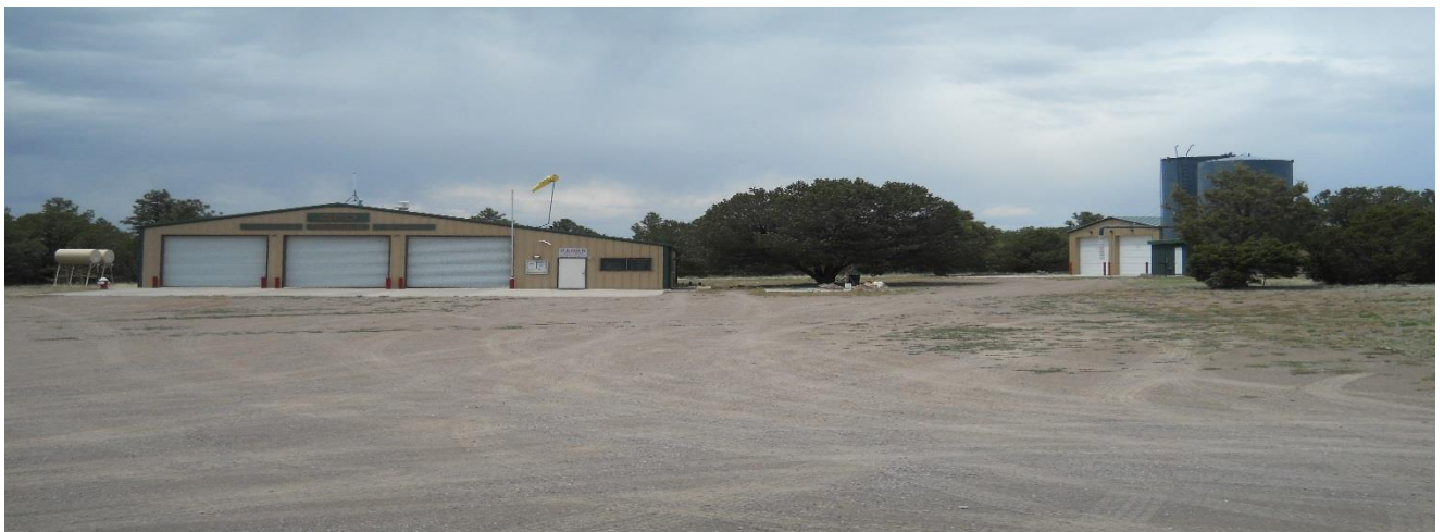
VFD station with helispot in driveway and 40,000 gallon water supply.
