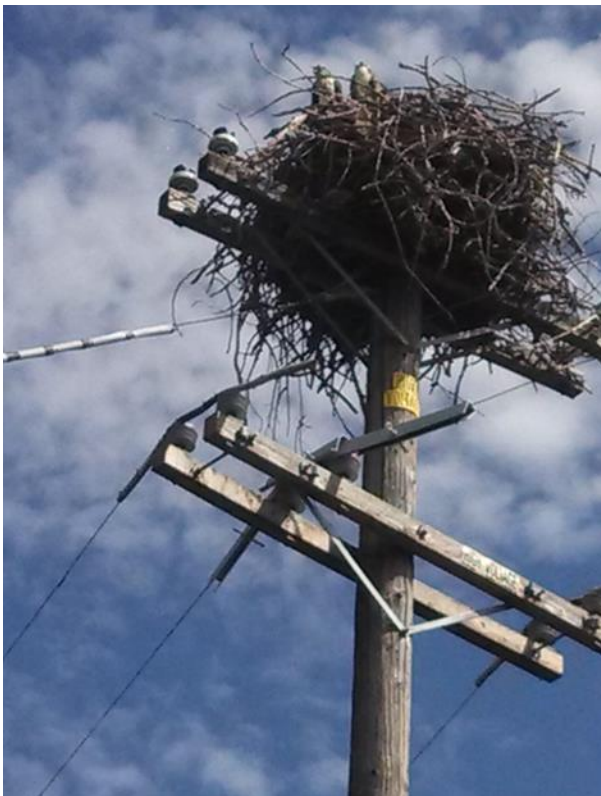
Figure 7.63. Bird nest above wires.
