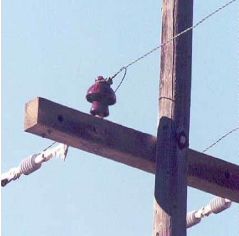
Figure 7.52. Typical crossarm insulator on a wooden mounting peg.
