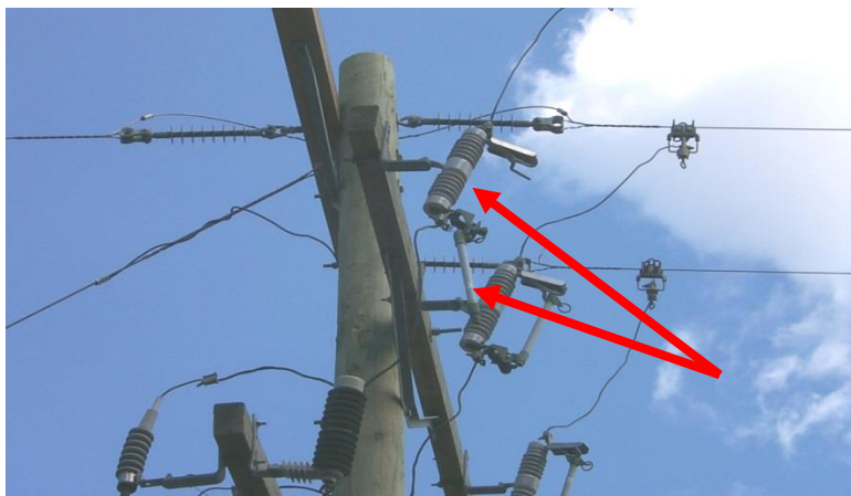
Figure 7.54. Solid blade disconnect.
