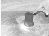
Missing spark arrestor
