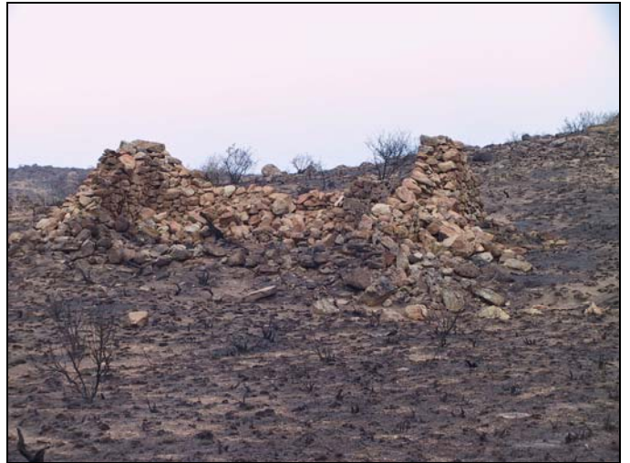
Tequero Dips stone building - note fire-blackened wall
