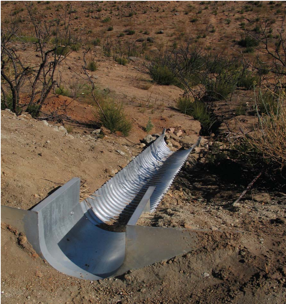
Metal Overside Drain. Page 118, Figure 70 of BAER Treatments Catalog (Dec. 2006)
