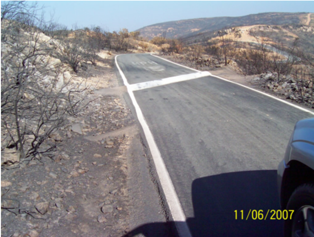
Example of typical asphalt bar, spur and outlet.
