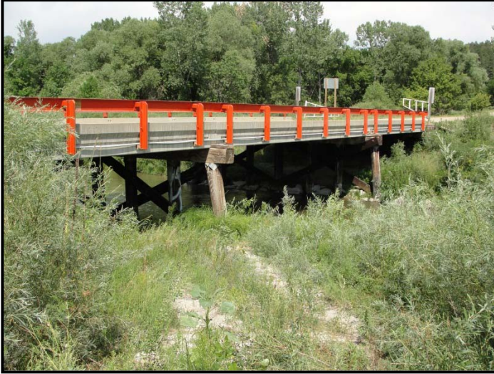
Beads Creek Bridge_Clearance is above bankfull levels.
