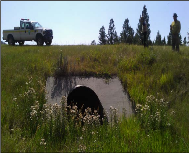
Highway 212 stream Crossing: Inspect and Maintain clean Culverts in response to expected Increased stream flows
