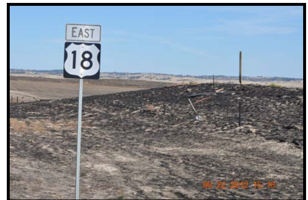
ROW Fence Destroyed Along US 18
