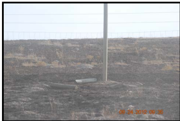
Buffalo Fence With Post Replaced
