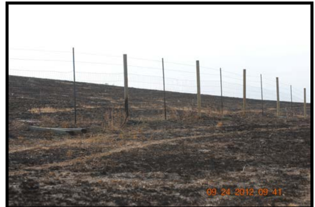
Buffalo Fence Damaged
